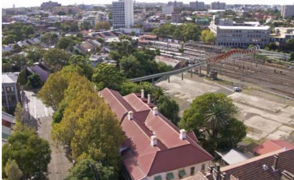
Figure H1.2 Aerial view looking south east
